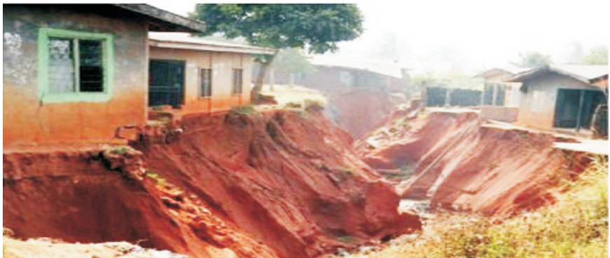
Fig 9: Gully Erosion Site in Delta State
