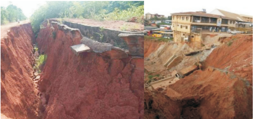
Fig 11: Landslides in Ubaha Nanka in Orumba North LGA of Anambra State
