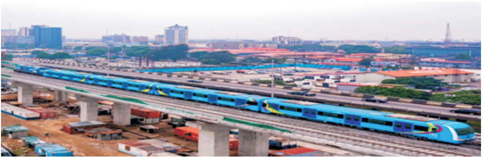
Figure 2: Improved Transport Infrastructure and Facilities- Lagos Rail Mass Transit (Vanguard, 2022).
