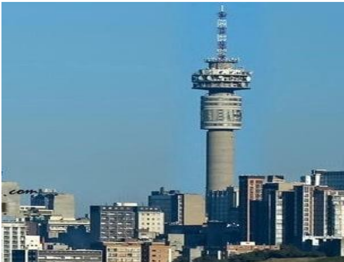
Figure 3: Sentech Tower in Johannesburg, South Africa Source: https://www.trip.com/review/sentech-tower-28682881-158136863
