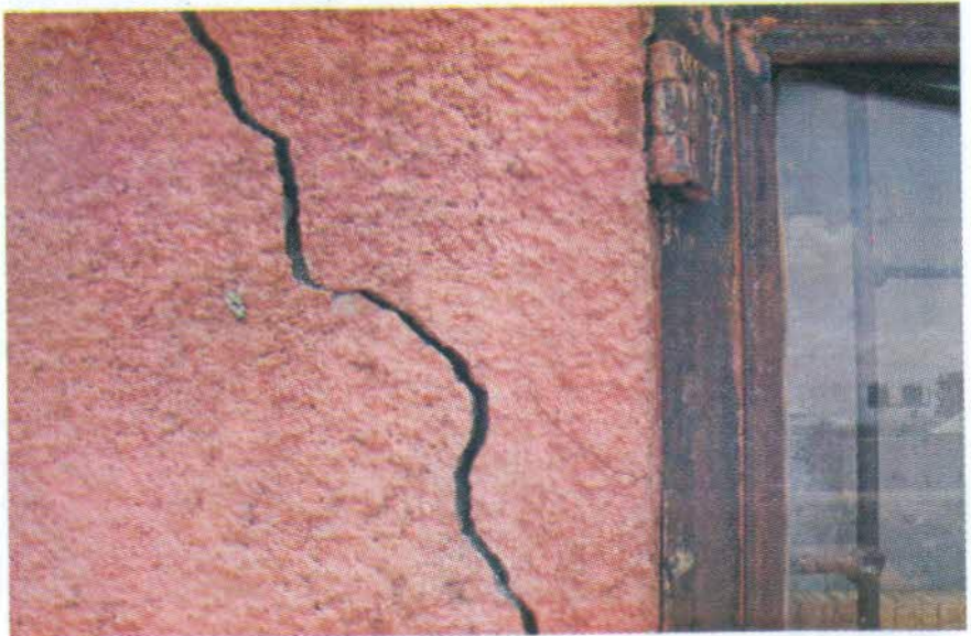
Figure 3: Cracked wall
