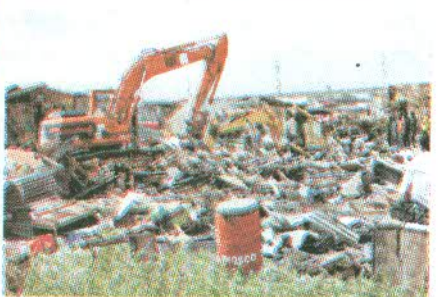
Plate XIX: Slum demolition in Kaduna
