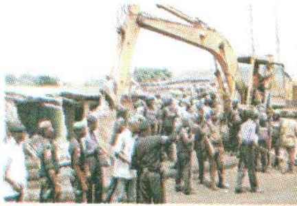
Plate XVI: Typical slum demolition in Lagos
