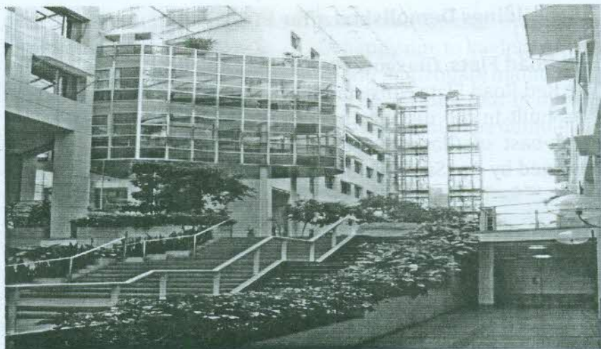
Plate 2.5 - SAS Building, Sweden Source: www.alamy.com
