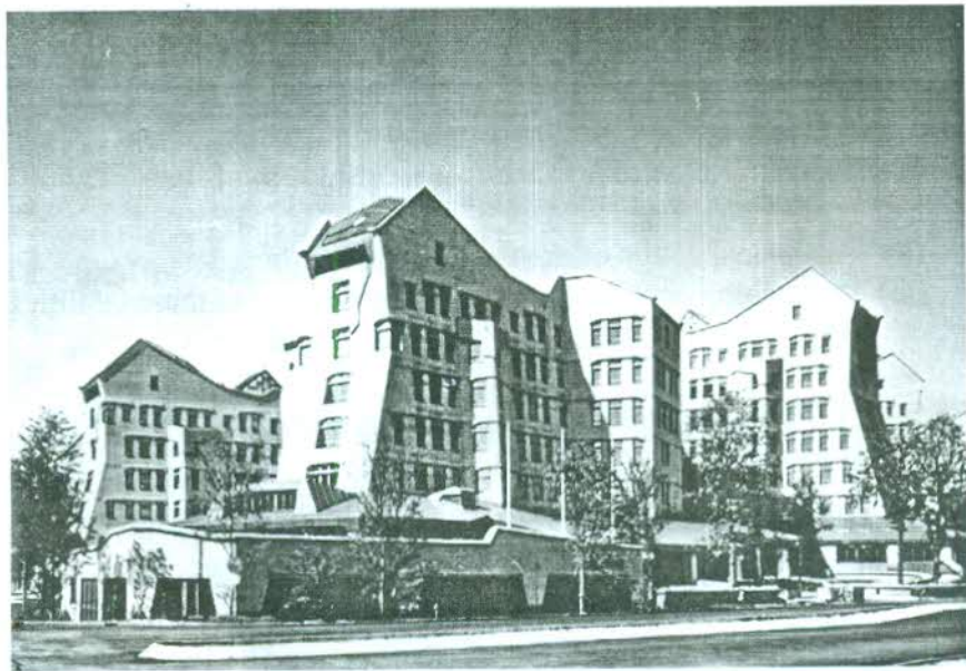
Plate 2.1 - NMB (now ING) Headquarters, Amsterdam, Netherlands Source: Architecture Guide (2018)
