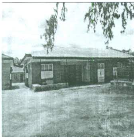
Plate 3.7 - Poor external image
