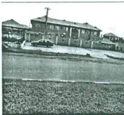
Plate 3.2 - Good access road
