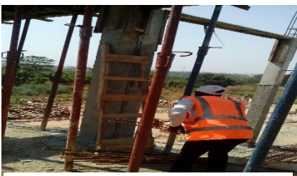
Figure 4.2 Iron Bender Working Under an Unsafe Area without Using PPE
