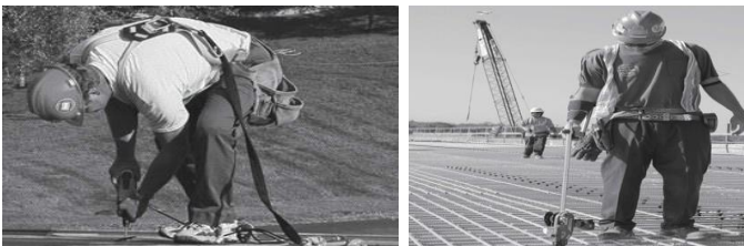
Fig. 4.5c: Bent posture and extended reach Fig. 4.5d: Tilt table brings work within reach
