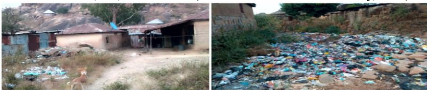
Plate IV: Building arrangements and the surroundings of informal settlements on Rukuba Road, Jos, Plateau State (Source: Researchers' field survey, 2021).
