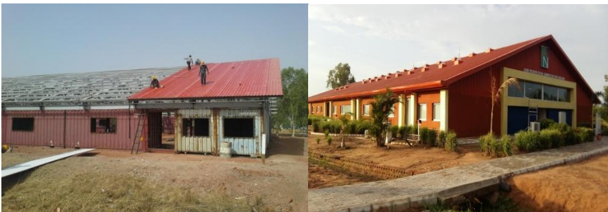
Plate I: Admin block 1 at the beginning and when completed
